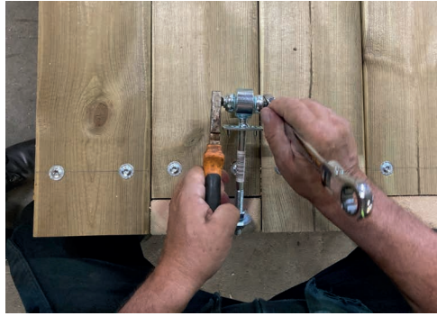
using a 17mm spanner slacken the nut
